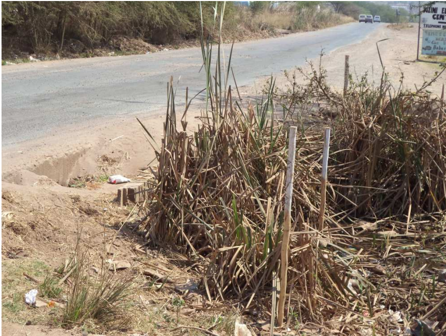
Figure 2.1: Existing Culvert at km 1.990 – Debris due to overtopping.
